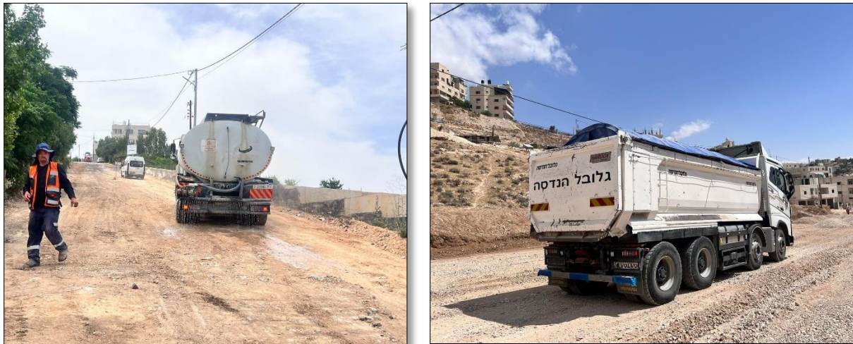
FIGURE 6: DUST CONTROL & COVERING CONSTRUCTION MATERIALS TRANSPORTED BY VEHICLES
