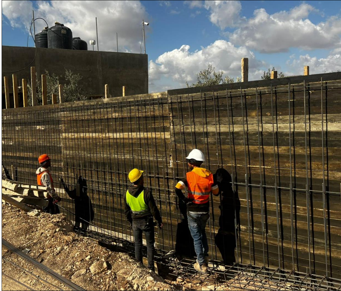
FIGURE 3: WORKERS WEARING PPEs
