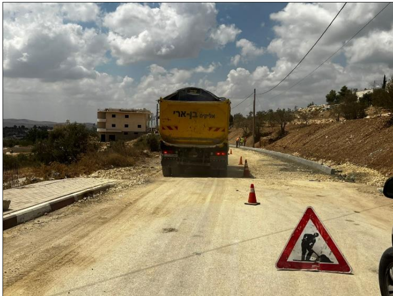
FIGURE 7: SAFETY AND GUIDING SIGNS IN THE PROJECT SITE & COORDINATION WITH POLICY
