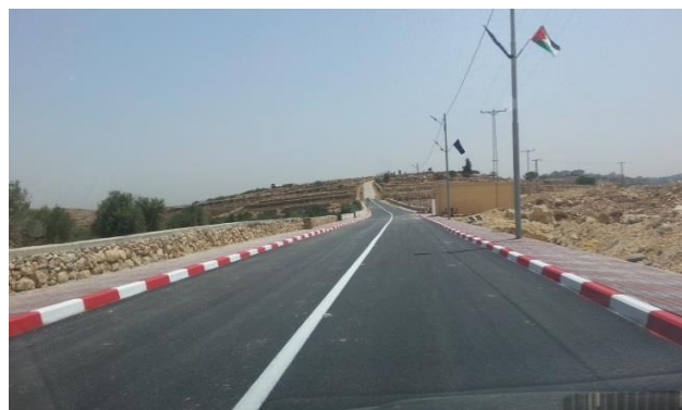
Rehabilitation of Internal Roads/ Um Al Lahim / Jerusalem
