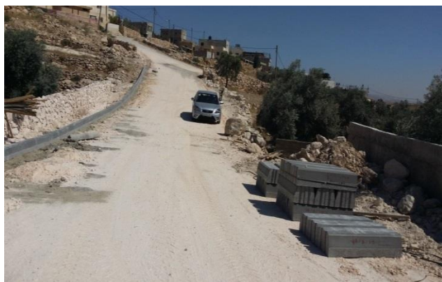
Rehabilitation of internal roads / Twaineh – Hebron
