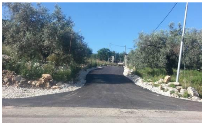
Rehabilitation of Roads / Izbet Al Tabeeb - Qalqilya
