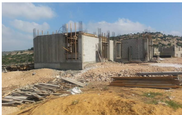
Construction of Service Center / Abdallah Al Younis - Jenin
