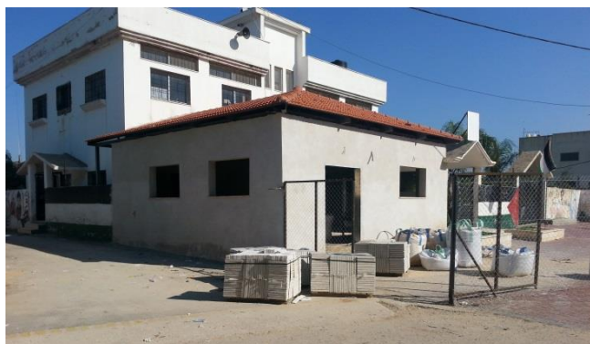
Finishing of Public Hall / Ezbit Al – Tabeeb / Qalqilia
