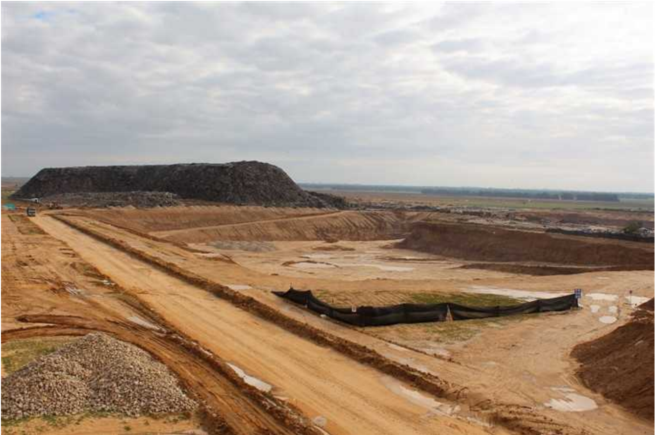
Image (1): Construction of Al-Fukhari Sanitary Landfill Rehabilitation of Existing Landfill in the Background
