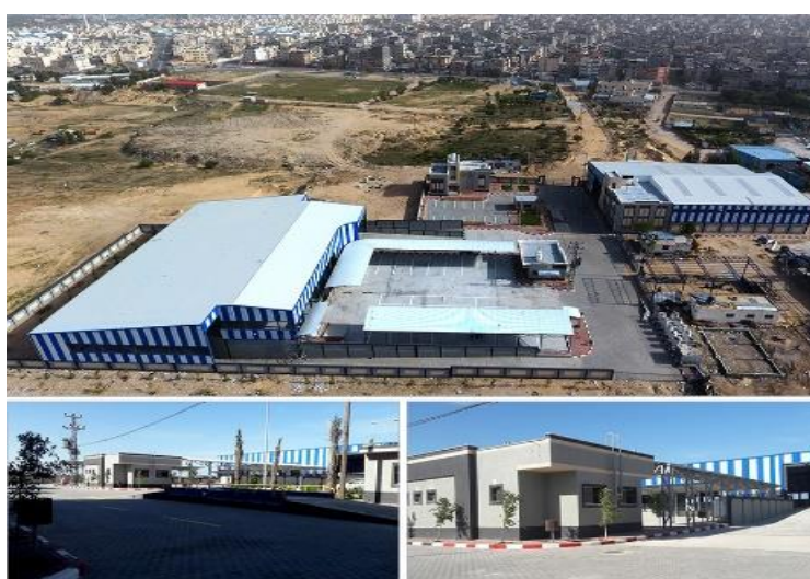
Rafah SW Transfer Station (December 2019)
