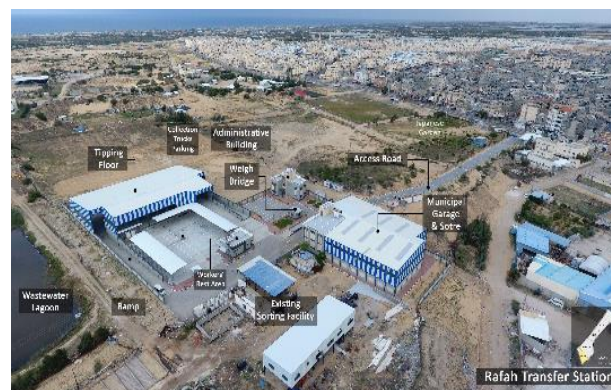
Rafah Transfer Station Compound (December 2019)
