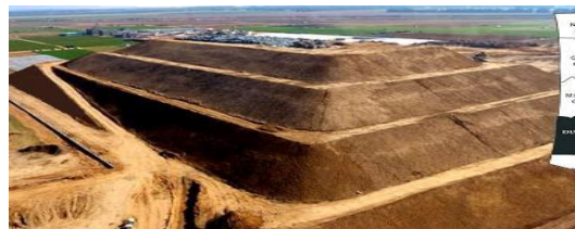
Al-Fukhari (Sofa) Existing Dumpsite partially closed prior to application of final cover and gas collection system.
