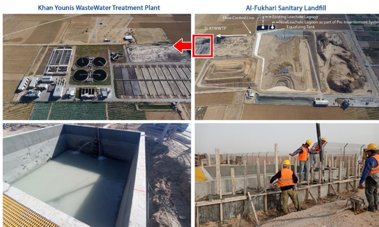
Leachate Pre-treatment System: Nov. 2022 → (TOP) Landfill and WWTP, (BOTTOM) construction activities of leachate pre-treatment facilities: equalizing tank, additional leachate lagoon, pressure lines infrastructure & civil works.
