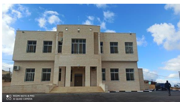
Image (1) and (2): A Building (Garage and Warehouse) for maintenance and operation for the Equipment
