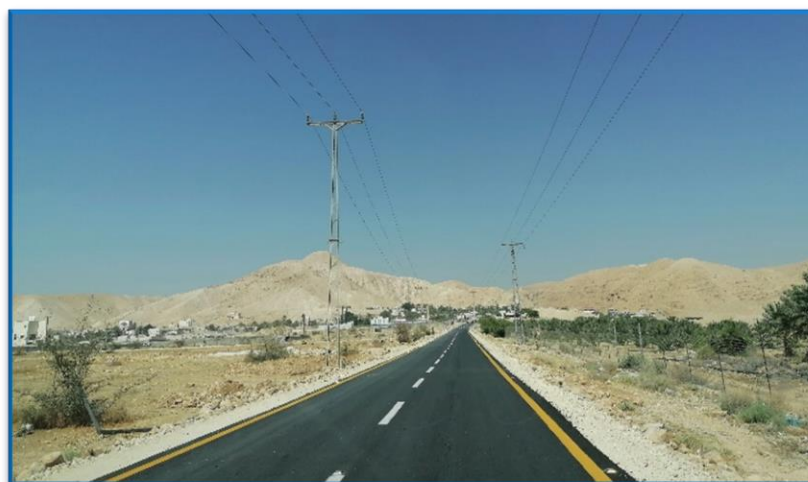
Municipal Garage road
