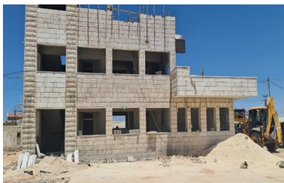
Construction of buildings
