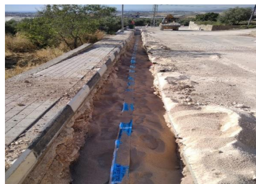
Construction of water distribution network
