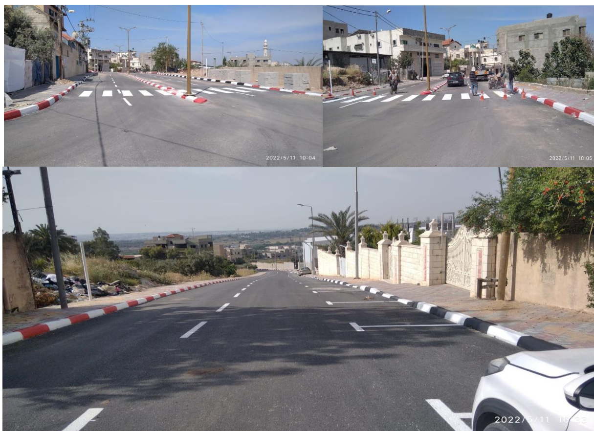
Rehabilitation of an Internal Road in Qalqilya
