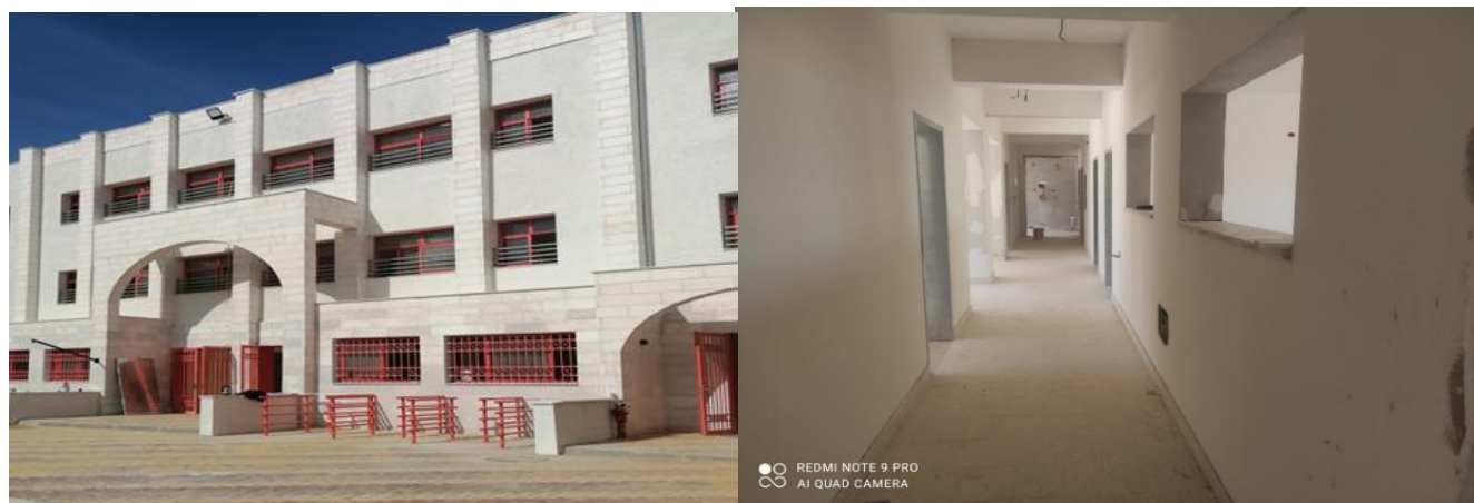
Continue the Construction of the Existing Haris Secondary Boys School
