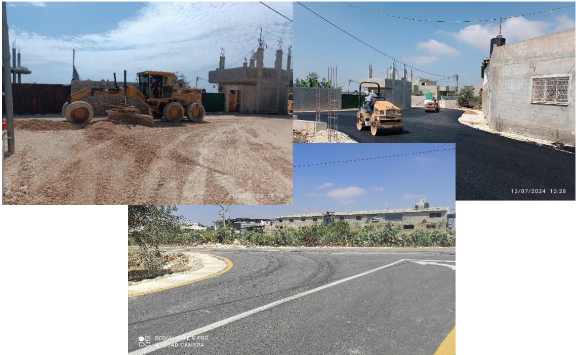
Rehabilitation of an internal road at Isla/Qalqilia
