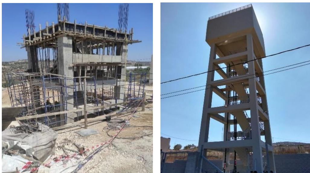
Construction 150 m3 Water tank and transmission pipeline – Al Mansoura
